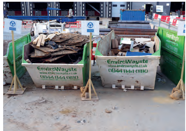
▲ Figure 3.6 Construction site waste being recycled in skips
