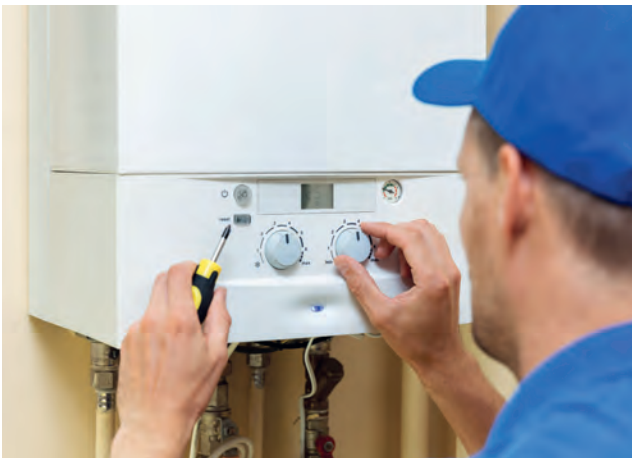
▲ Figure 3.17 Retrofit installer fitting an energy-efficient boiler
