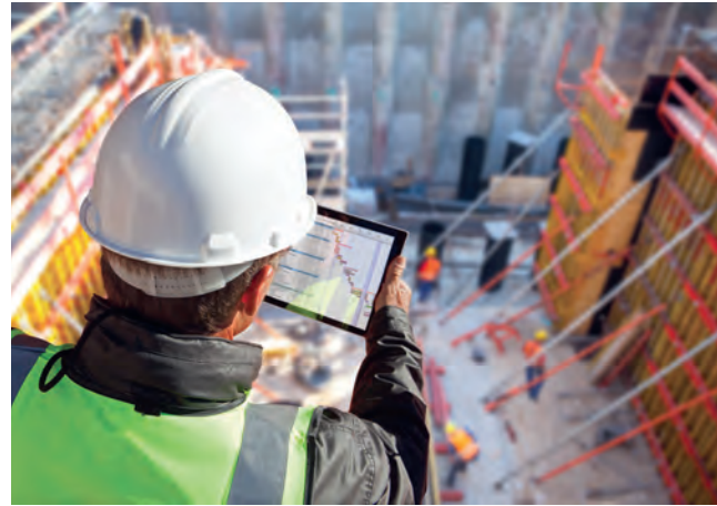
▲ Figure 3.23 A site manager monitoring progress against the programme of work
