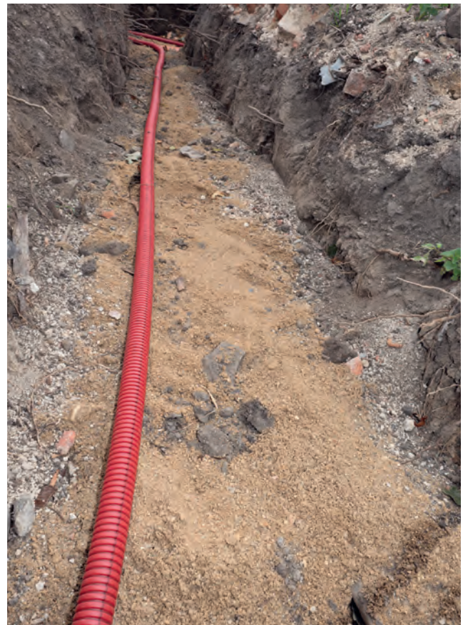
▲ Figure 3.11 Services being connected
