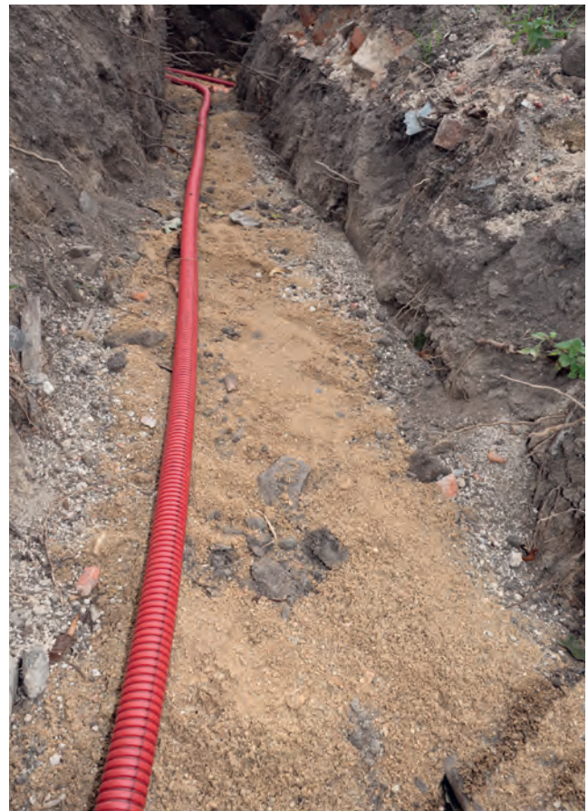
▲ Figure 3.11 Services being connected
