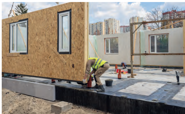
▲ Figure 3.13 A cassette being lifted into position on site
