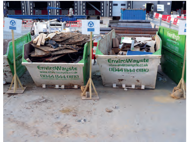
▲ Figure 3.6 Construction site waste being recycled in skips
