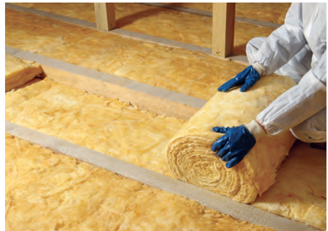
▲ Figure 3.4 Loft insulation
