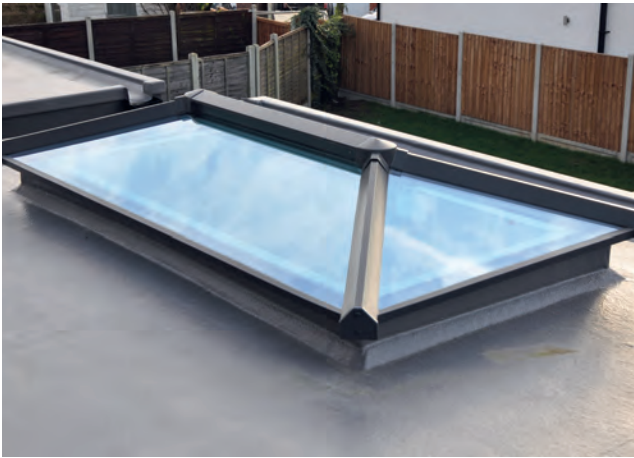
▲ Figure 3.14 Natural light entering a building through roof lanterns
