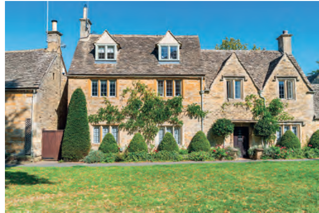
▲ Figure 3.10 This stone house in the Cotswolds, built with local materials, is an example of vernacular construction
