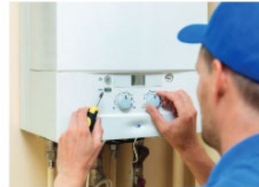
▲ Figure 3.17 Retrofit installer fitting an energy-efficient boiler
